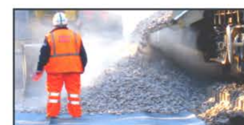
Fig. 6: dust production from ballast transport. Credit: Network Rail
