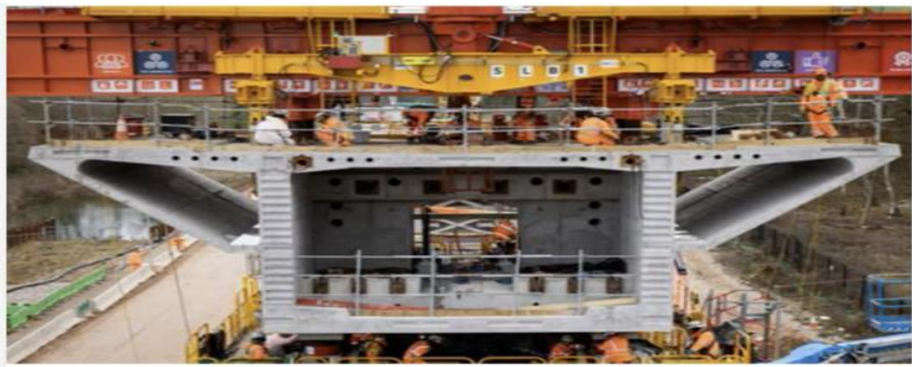
UK's longest rail viaduct – HS2 Colne Valley Viaduct
